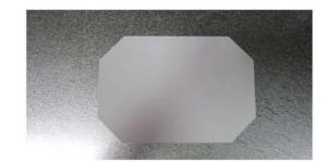
Closely cut duct around the perimeter of template and remove portion of duct. We recommend using a small jig-saw blade #30076 or conventional sheet metal nibbler. You may want to drill a pilot hole in the 4 corners to make cutting easier.
