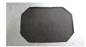
Center and place Access Armor Duct Door into opening, being sure that all D-ring fasteners are in the "open" / counter-clockwise position. Note: De-burring perimeter of duct opening is recommended to ensure proper fitting for access door and to reduce risk of injury.
